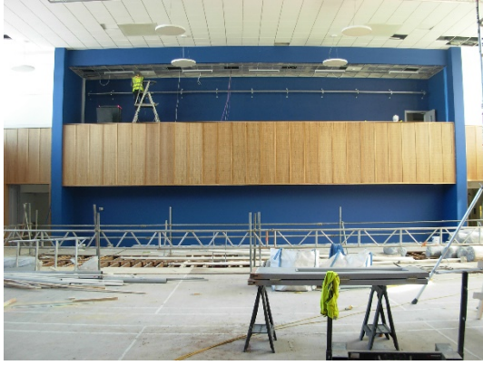
View from stage back to the Technical Gallery. New solid oak floor to be laid
