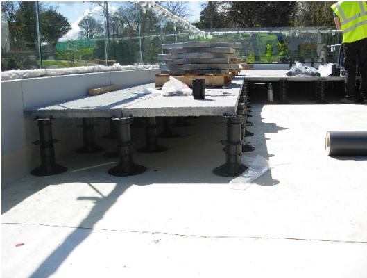
Second floor – precast pavers being installed on roof terrace
