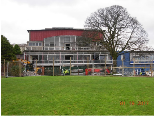
The southern elevation from Castle Gardens
